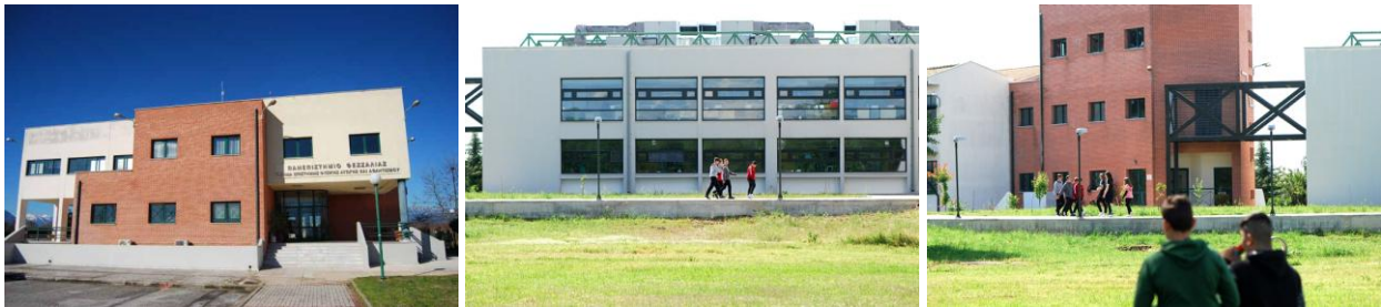
Part of the TEFAA facilities.
